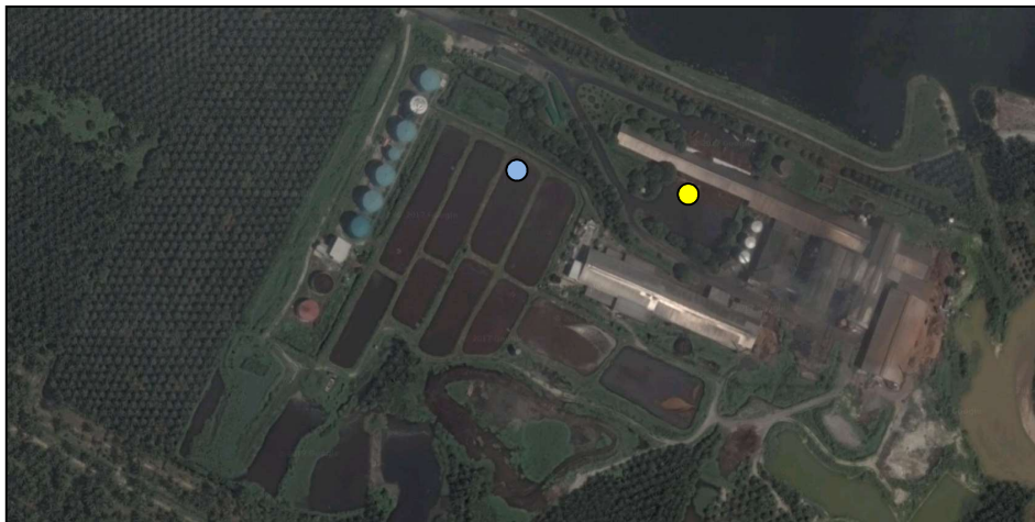
Fig. 3. The anaerobic tank digesters as part of the palm oil mill effluent treatment at Mill C. On-site odour assessment was performed nearby the anaerobic ponds (●), while odour samples were collected from the cooling pond (●, with an estimated size of 90 m x 45 m = 4050 m 2 )
